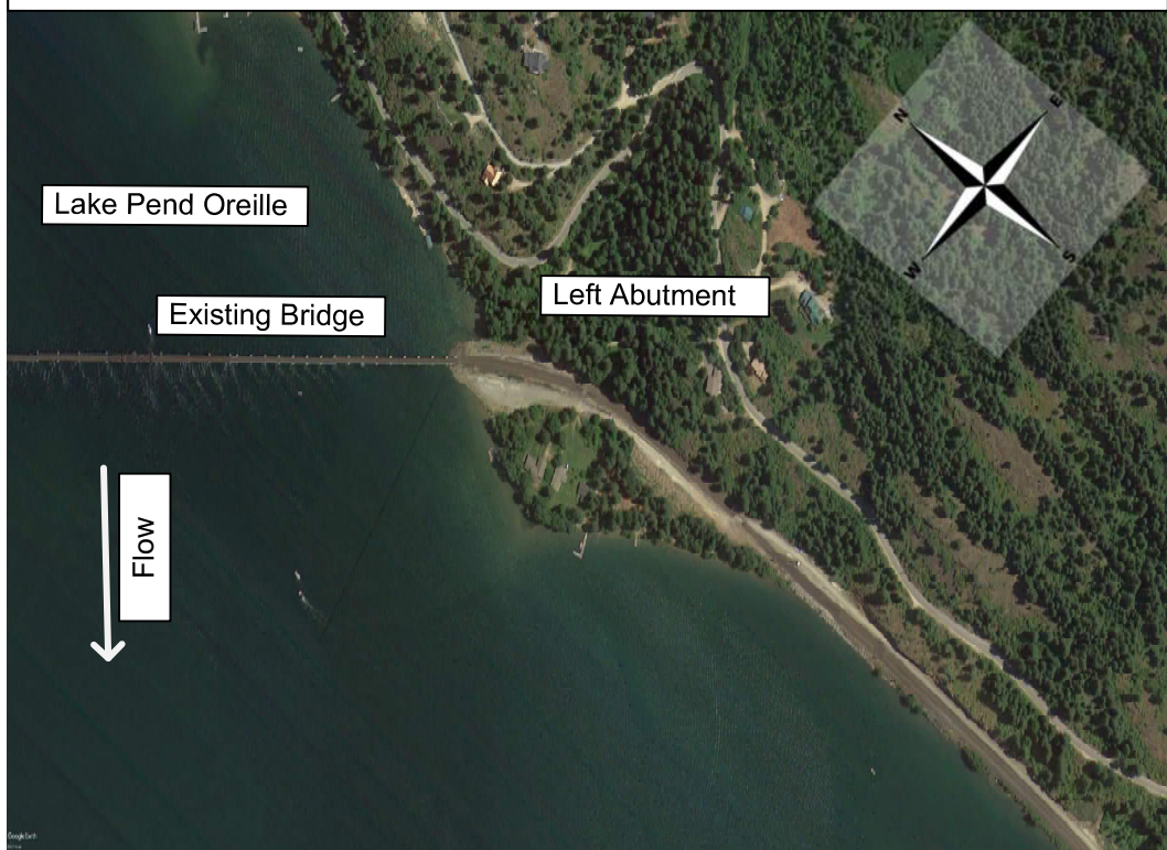
Photograph 2 – Aerial View of Existing Bridge on Lake Pend Oreille
