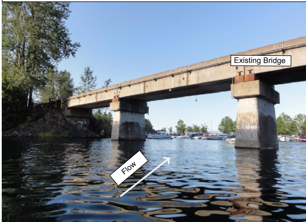
Photograph 2 – Left abutment of Existing Bridge looking Downstream (northeast)
