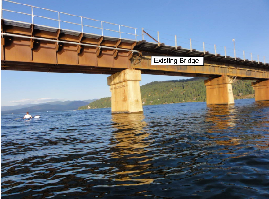
Photograph 9 – Existing Bridge Concrete Piers on Lake Pend Oreille
