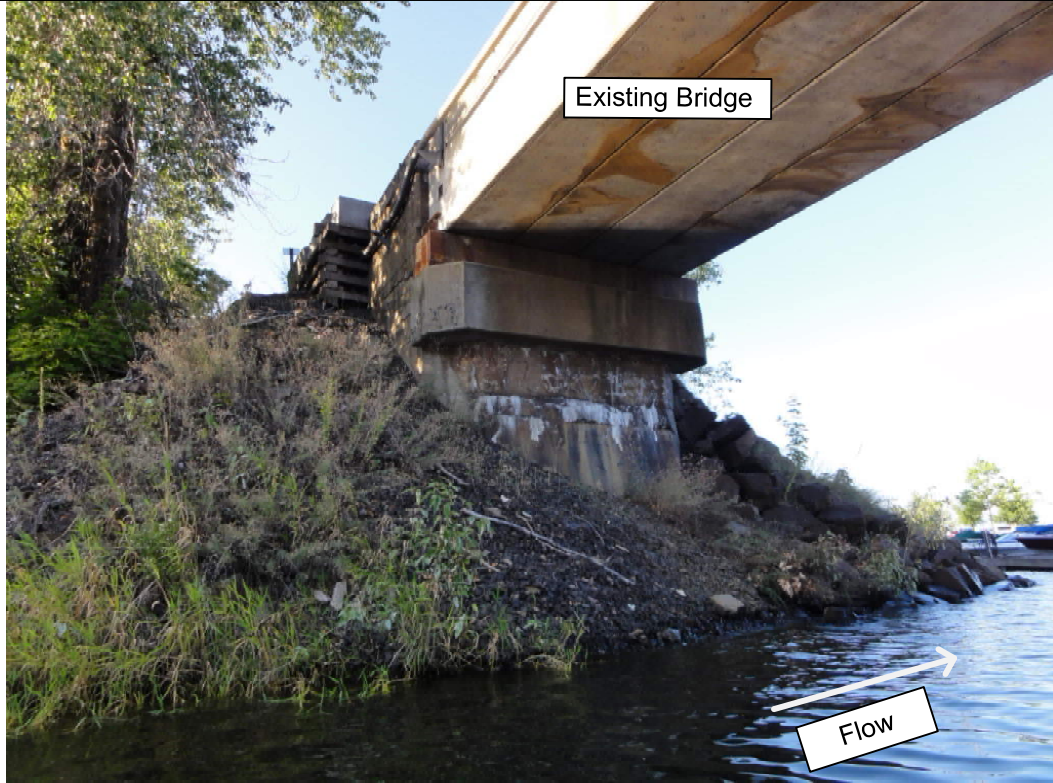
Photograph 5 – Left abutment of Existing Bridge looking north
