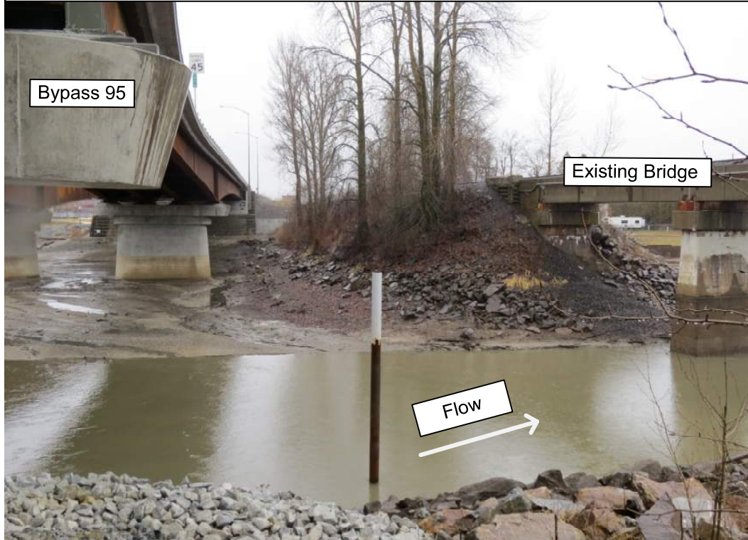
Photograph 4 – Left abutment of Existing Bridge looking north
