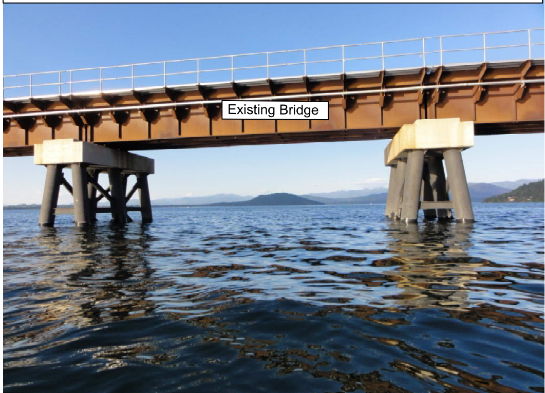
Photograph 10 – Existing Bridge Battered Piers on Lake Pend Oreille
