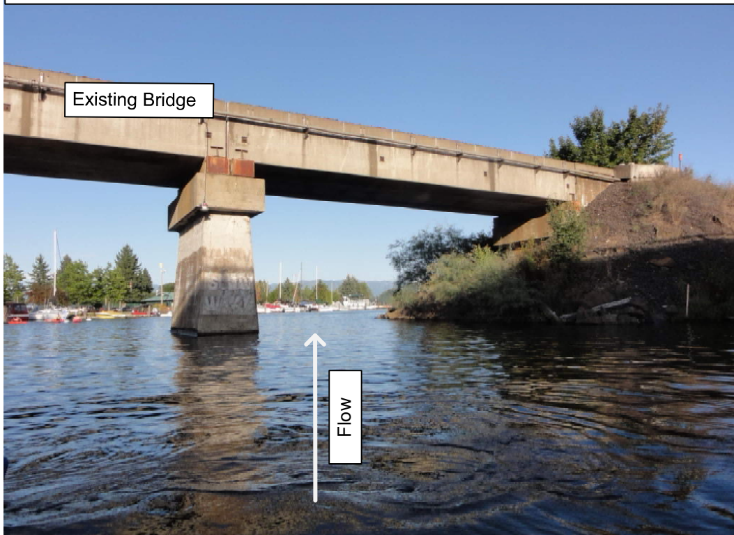
Photograph 6 – Right abutment of Existing Bridge looking Downstream (southeast)
