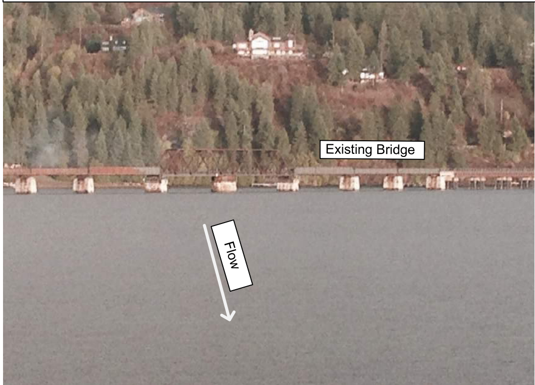
Photograph 8 – Existing Bridge Truss on Lake Pend Oreille looking Upstream (east)
