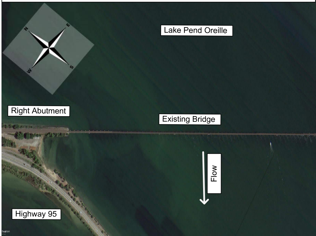
Photograph 1 – Aerial View of Existing Bridge on Lake Pend Oreille
